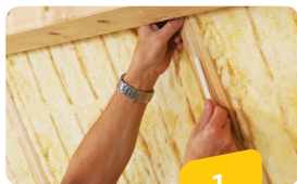
Attaching the XtraFix to a hard surface
