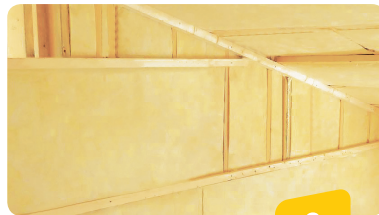
Internal Thermal Bridge Blocking
