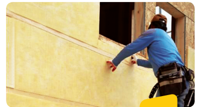
External Thermal Bridge Blocking
