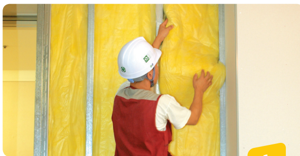
Safe Wall Installation
