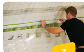
Attaching of the film joint by XtraTape
