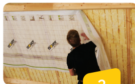
Attaching XtraSafe on XtraFix
